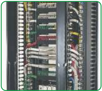
Polycarbonate / ABS finger On front and back side
